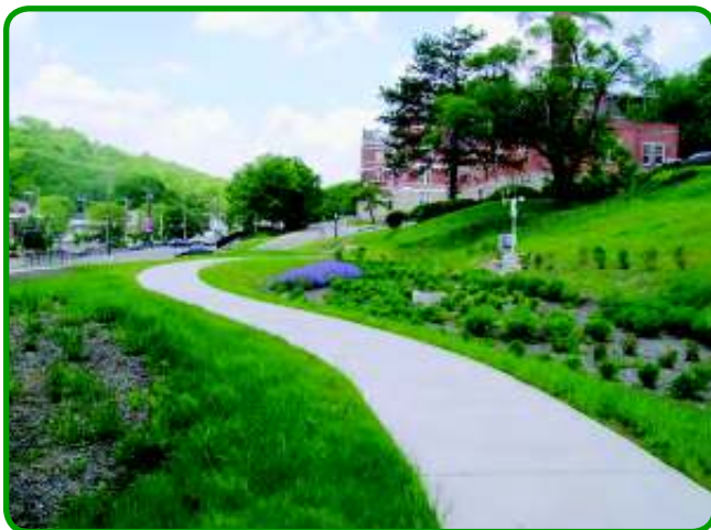
Rain gardens at the HUD-owned St. Francis Senior Apartments replaced excess pavement to reduce stormwater runoff. A monitoring station, pictured at right, measures runoff levels. Photo courtesy of EPA.
