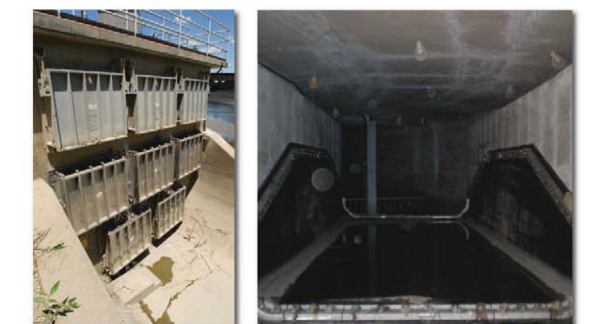
Example RTC facilities
