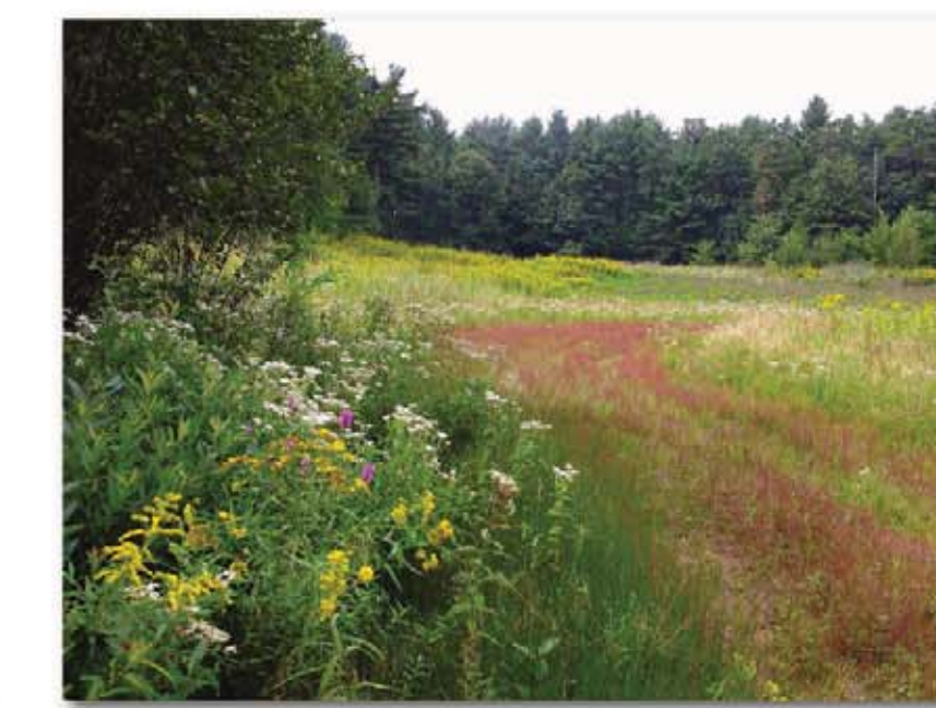
Stormwater Detention Basin
