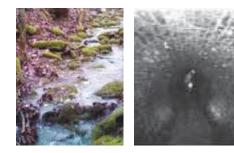
Above: A comparison between a natural stream and a buried stream enclosed in a brick combined sewer from the 1800s. Left photo by Robert Hawley, right photo from the Lick Run Master Plan, 2012
