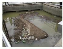
The second project uses a pair of rain gardens installed at the St. Francis Apartments. The rain gardens are designed to reduce the amount of stormwater runoff reaching the Lick Run sewer system, and to improve water quality by filtering parking lot runoff.
