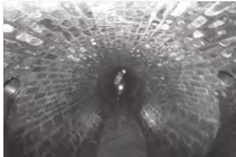
Brick sewer from the 1800s
