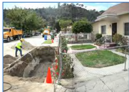
Constructing green infrastructure features in locations with poor sidewalks improves water quality and pedestrian facilities. (City of Los Angeles 2010, www.lastormwater.org )
