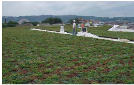
Green roofs not only detain stormwater – they also insulate buildings and create habitat for birds and insects.
