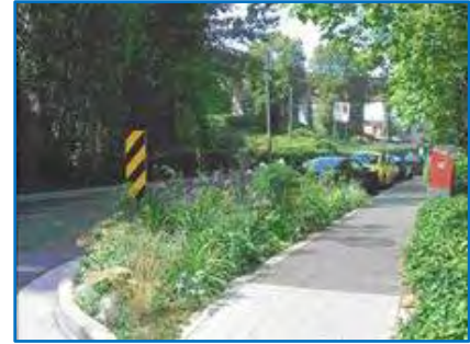
An example of a "green street" with bioretention (Low Impact Development Center 2011)
