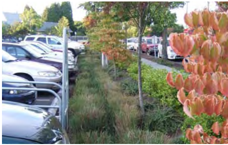
Bioswales are designed to capture stormwater, filter out pollutants, and reduce flooding.
