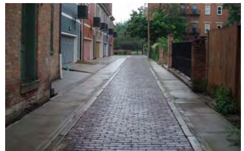
Pervious pavers help rainwater seep into the ground, thereby helping to reduce stormwater runoff.
