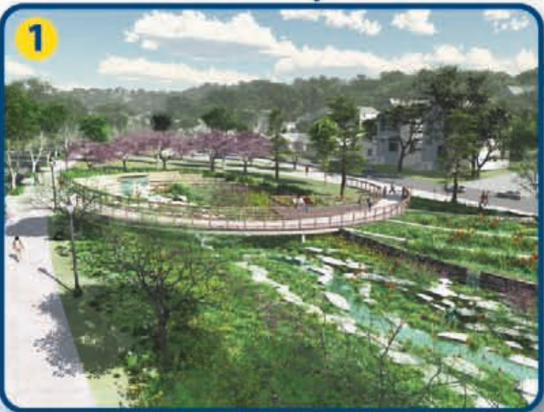
(Looking Northwest) This image depicts the daylighting of stormwater into the proposed urban waterway. The proposed urban waterway will contain water quality features (limestone rock) and a well-vegetated riparian edge. Rain gardens will help to intercept stormwater from Queen City Avenue and direct it into the waterway. Lighting is included to ensure the multi-purpose trail on Westwood is well lit and safe for pedestrians.
