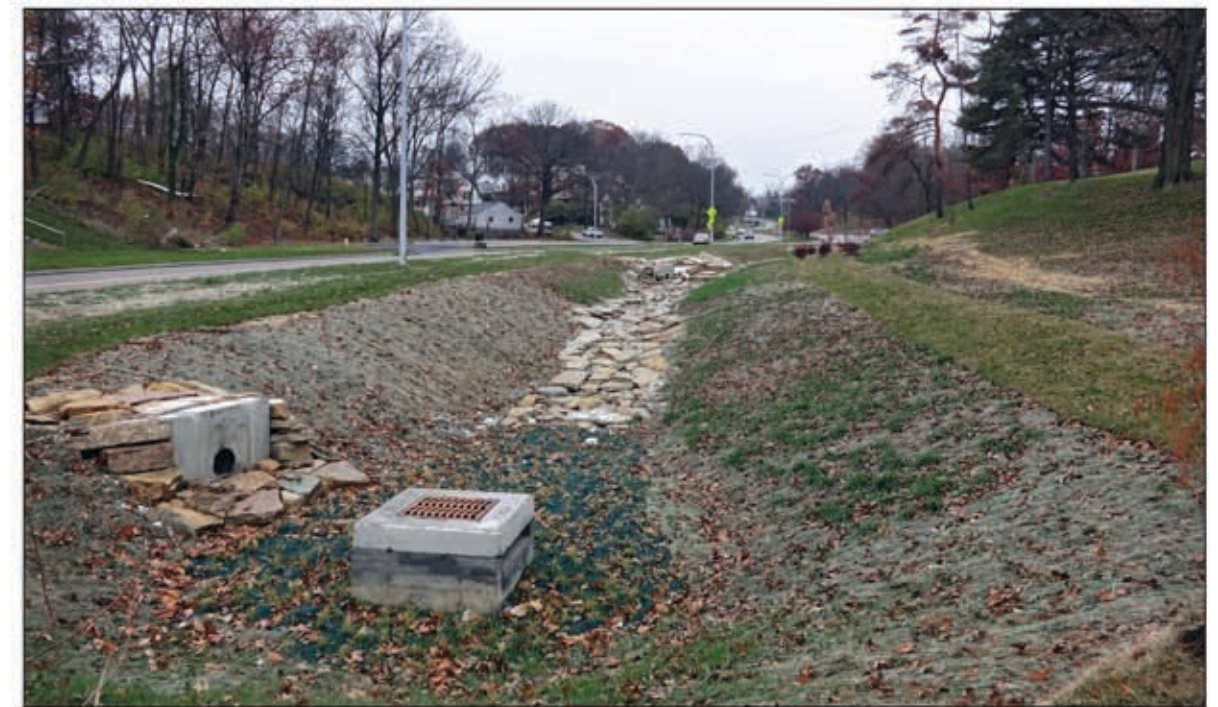
Completed bioswale during dry weather
