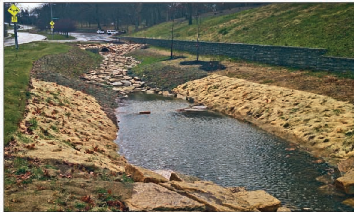
Completed bioswale during rain event
