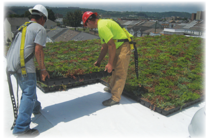
Taft Information Technology High School: A 32,000-square foot shallow vegetative roof was installed on the roof of the Taft Information Technology High School.
