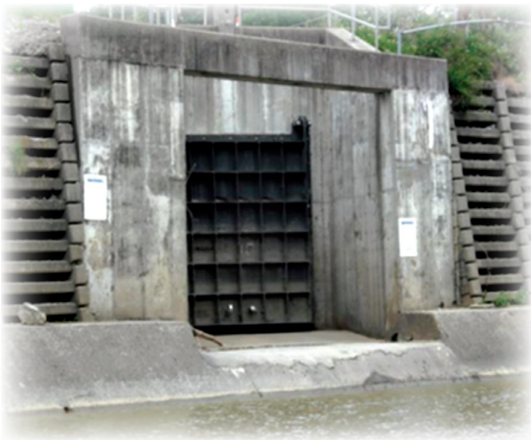
CSO 24, Ludlow Run Regulator, averages 318 million gallons of overflow a year, the highest of all the CSOs.
