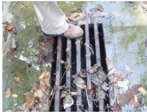
Invert Grates Connect Channel to Interceptor
