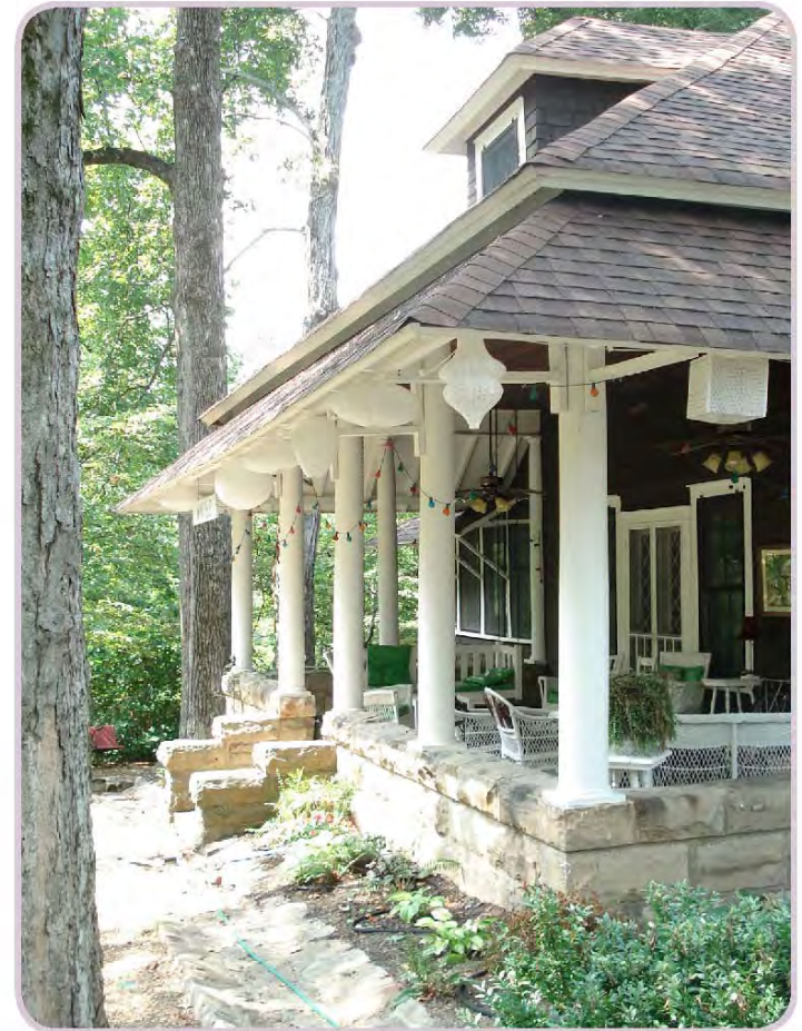
T3 - Gutter - Monteagle, TN
