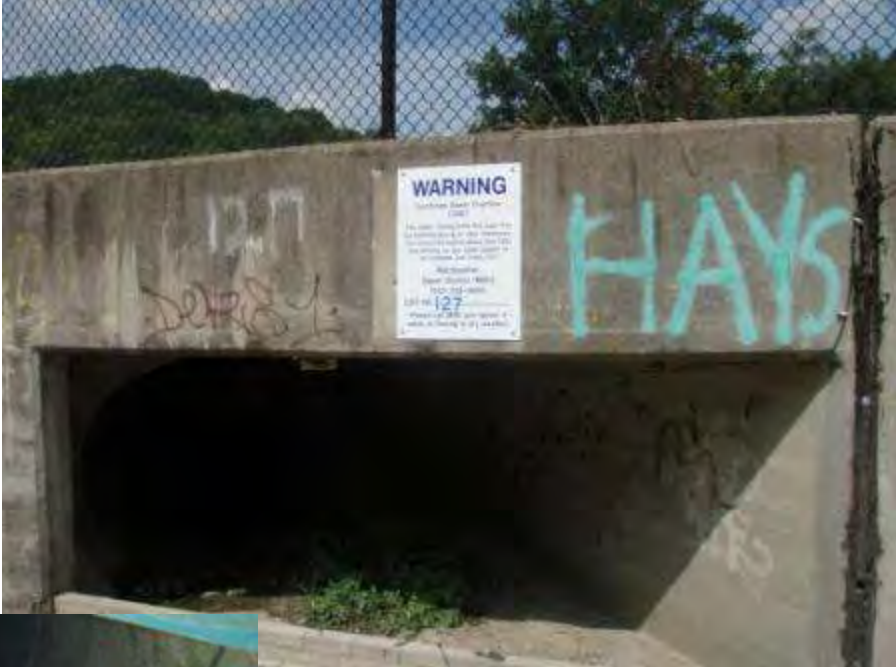
CSOs Discharge into Channel
