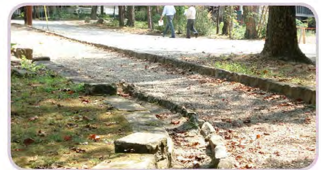
T3 - Gutter and Curb - Monteagle, TN
