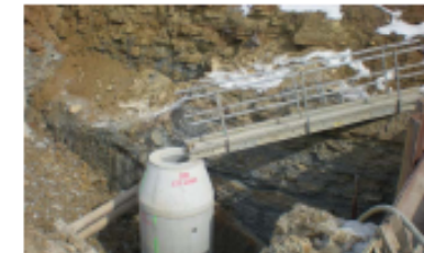
New MH #21 on north side of Westwood Northern Blvd.
