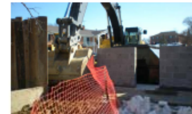
Excavation of Diamond Oaks Pump Station holding tank
